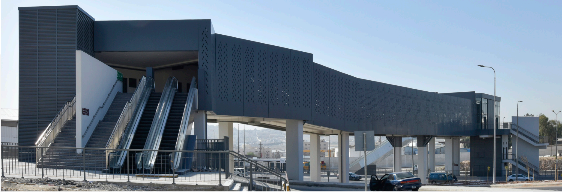
Amman-Zarqa bus rapid transit (PK5) Hashemeyeh Station, 2023.
