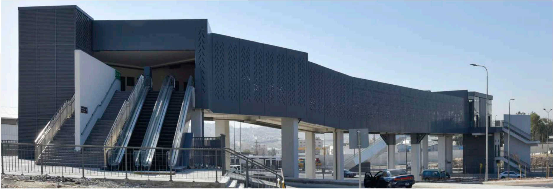
Amman-Zarqa bus rapid transit (PK5) Hashemeyeh Station, 2023.
