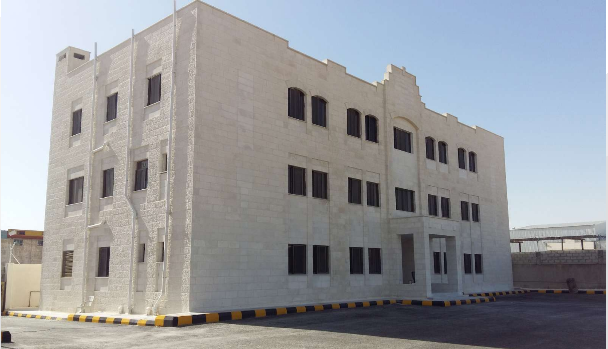
Construction of Zarqa Free Zone Civil Defense Center, 2016.
