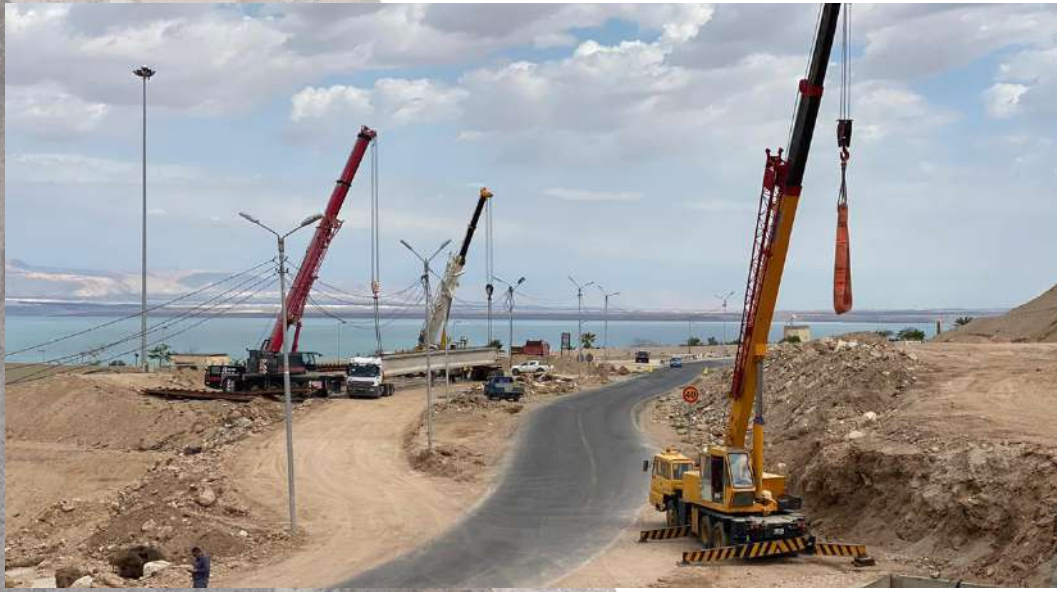
Protection Works For Bridges Along Dead Sea – Ghor Hadetha –Road –Package 2, 2021.
